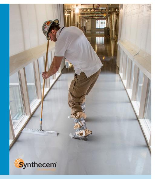
For projects that you can only afford to do once. **Platform L3** quickly fixes uneven or damaged floors with minimal prep. Powered by **Synthecem™** technology, it provides a smooth, durable surface, ready for flooring in as little as 12 hours.
